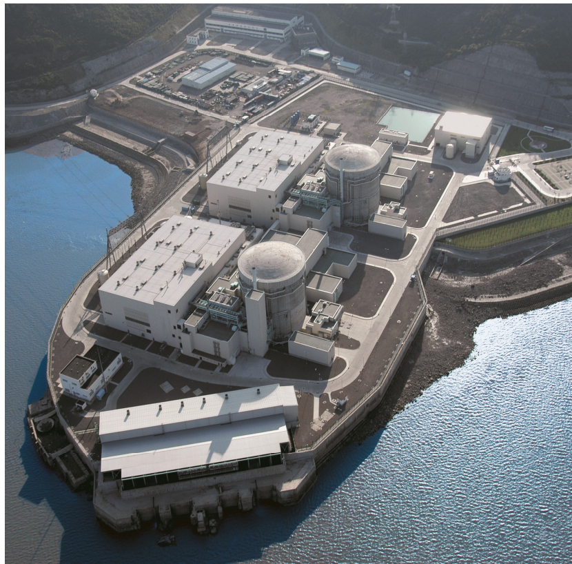
Figure 5 Qinshan CANDU Reactors in Haiyan, China
