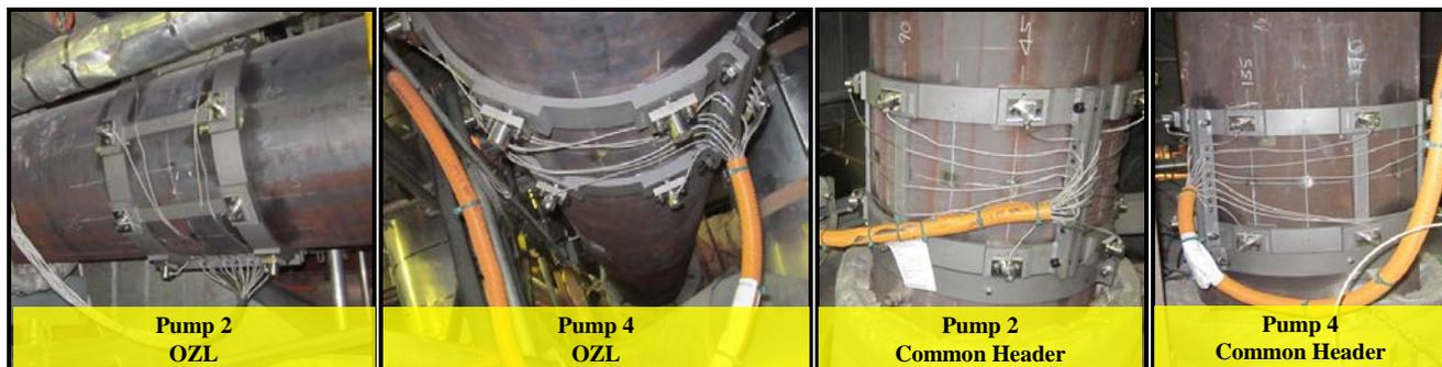
Figure 6 Installation on Pump 2 and Pump 4 OZL and Common Header pipes
