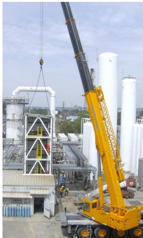
Figure 7 Complete Columns Module being Erected
