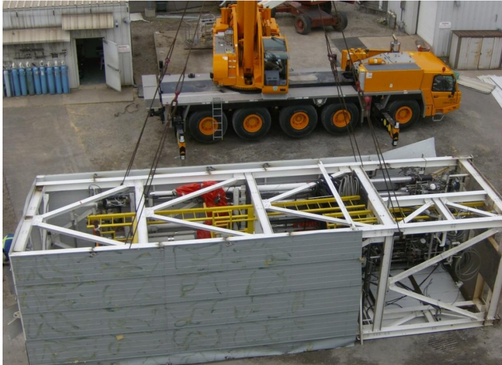
Figure 6 Complete Columns Module being prepared for Transportation
