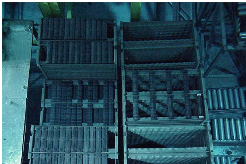
Figure 2 Storage Trays in Spent Fuel Bay
