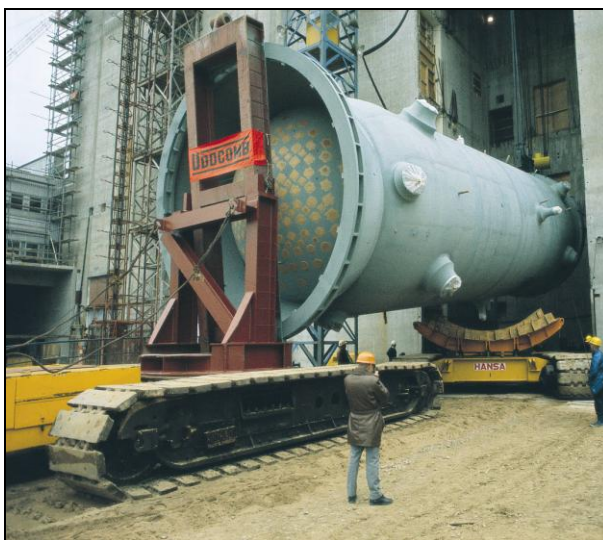
Figure 6. Installing one of the two RPVs (BWR) at the Barsebäck site in the 1970s.
