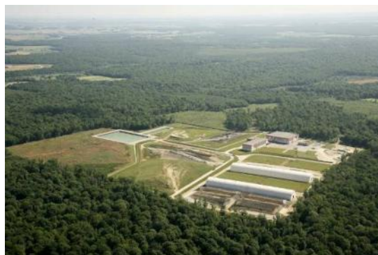
Figure 14 : general view of Morvilliers disposal facility
