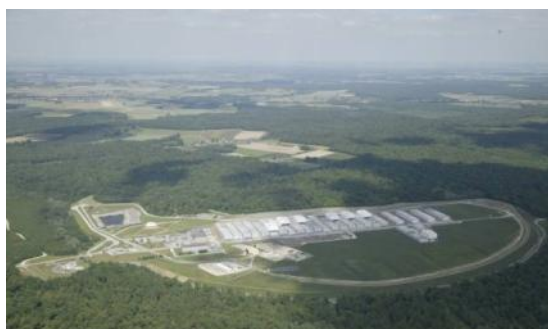
Figure 10 : centre de l'Aube disposal facility
