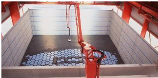
Figure 12 : grouting of metallic packages in a disposal vault
