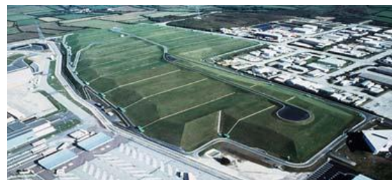
Figure 7 : Centre de la Manche capping system
