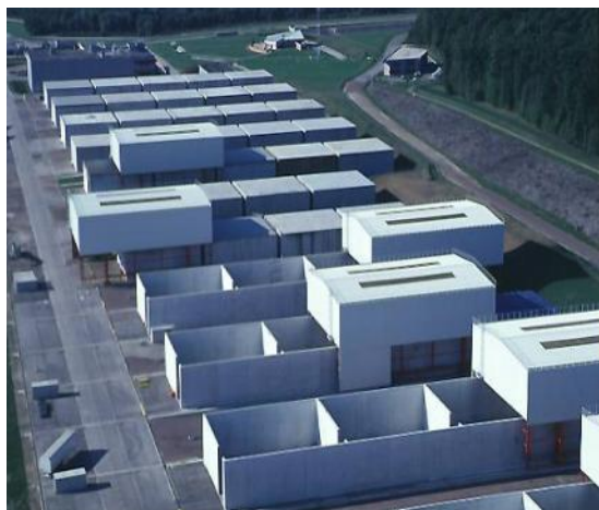
Figure 11 : disposal vaults at Centre de l'Aube
