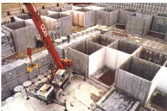
Figure 3 : disposal operations in monolithic cells (1985)
