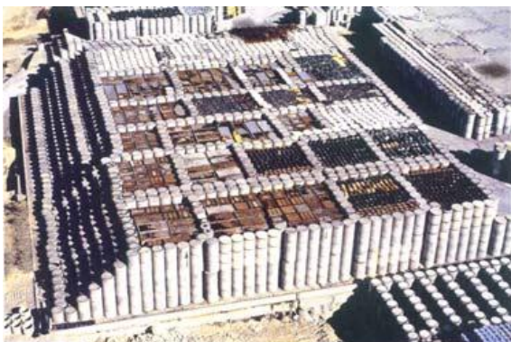
Figure 4 : above ground disposal structure (1988)
