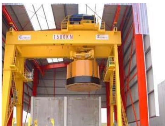
Figure 13 : disposal of a reactor vessel head
