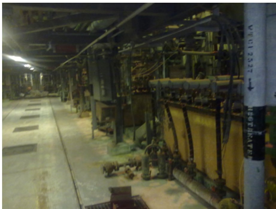
Figure A-4: NECSA Uranium Conversion Facility Awaiting Decommissioning.
