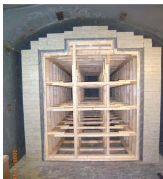
Clay Blocks in Place
