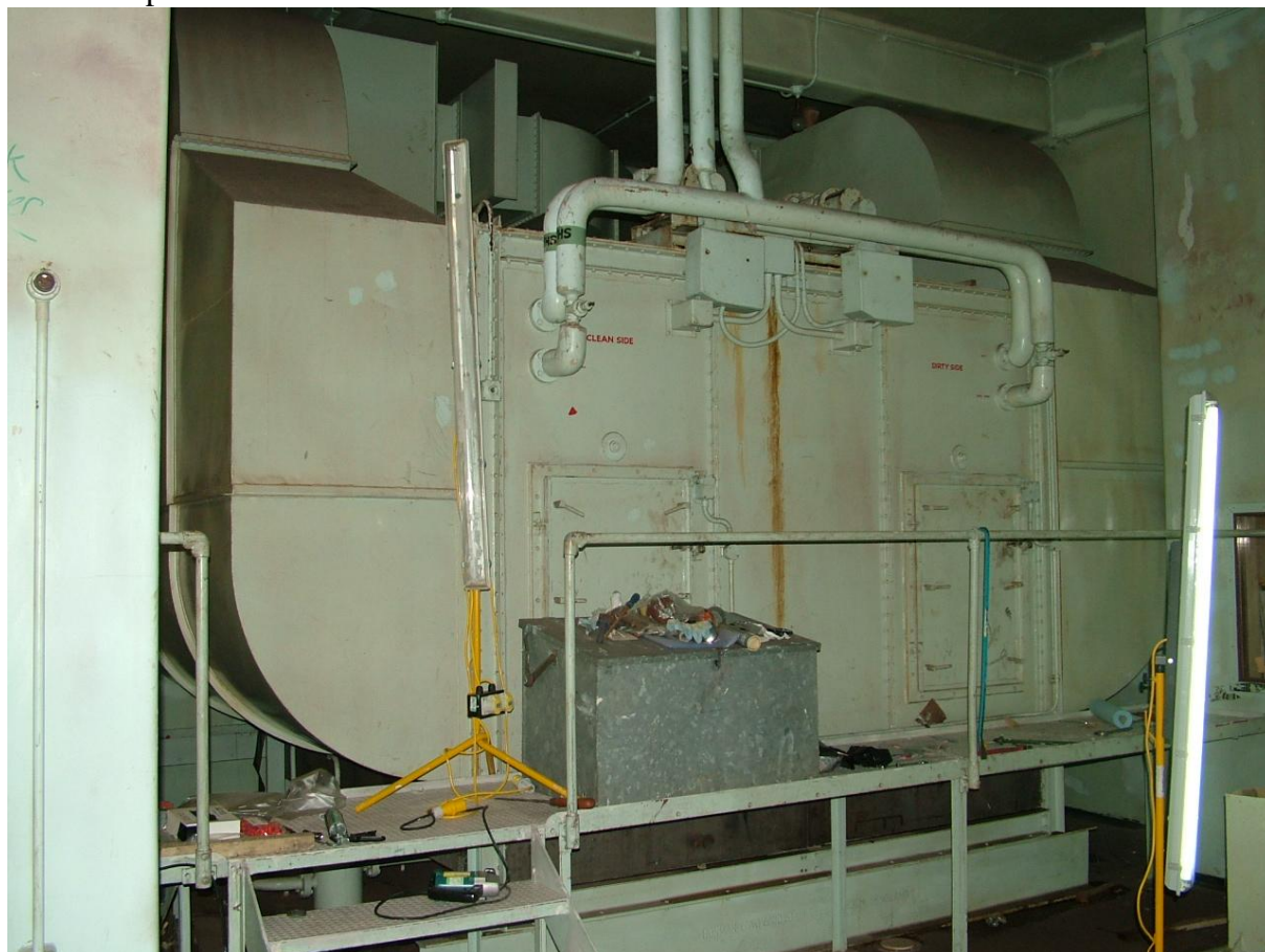
Figure 7: A View of the Precipatron Unit before Strip-Out
