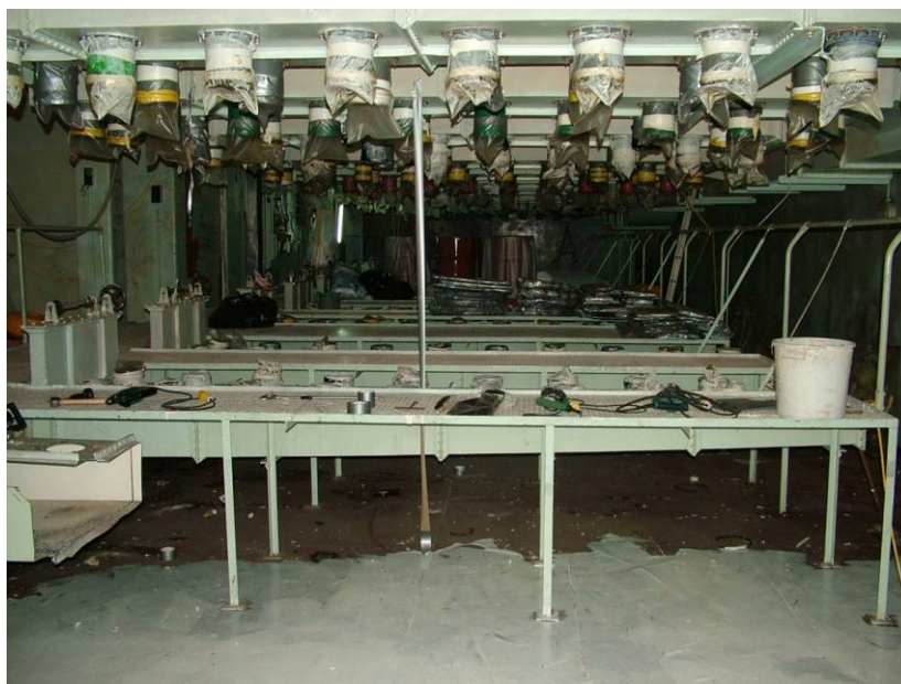
Figure 6: A View of the UFMA Extract Filter Bank during Strip-Out
