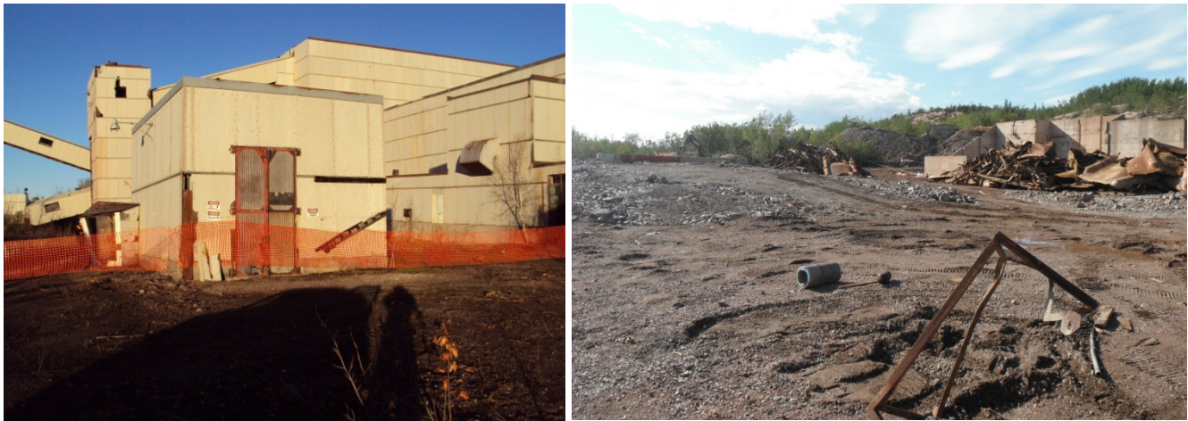
Figure 6. Before (left panel) and after (right panel) photos of the demolition of the Gunnar Mill Complex following remediation efforts in 2011 at the Gunnar Mine Site.
