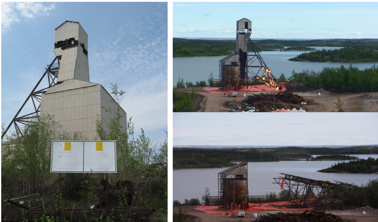
Figure 7. Before (left panel) and after (right panels) photos of the demolition of the Gunnar Headframe following remediation efforts in 2011 at the Gunnar Mine Site.
