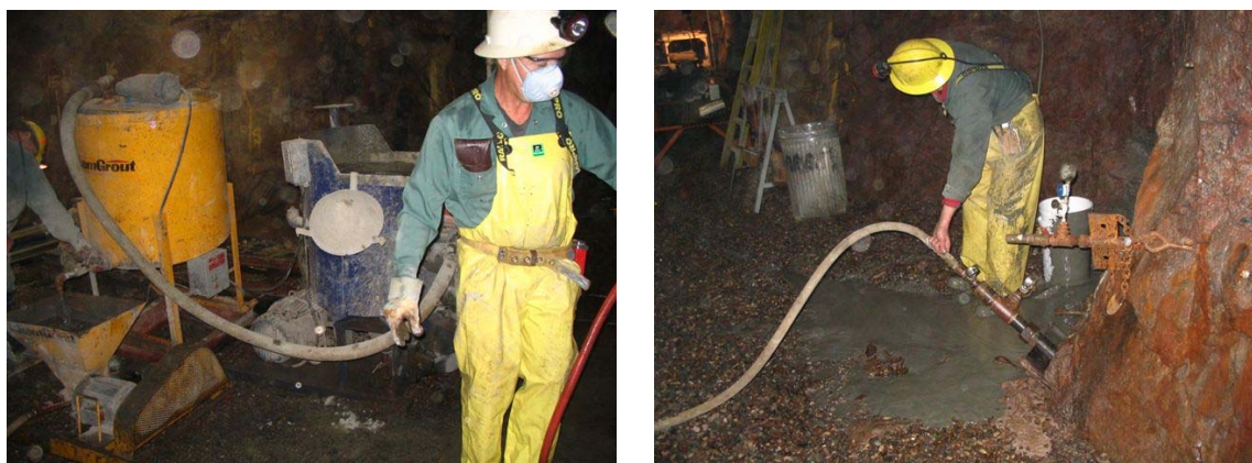
Figure 3. Borehole grouting.
