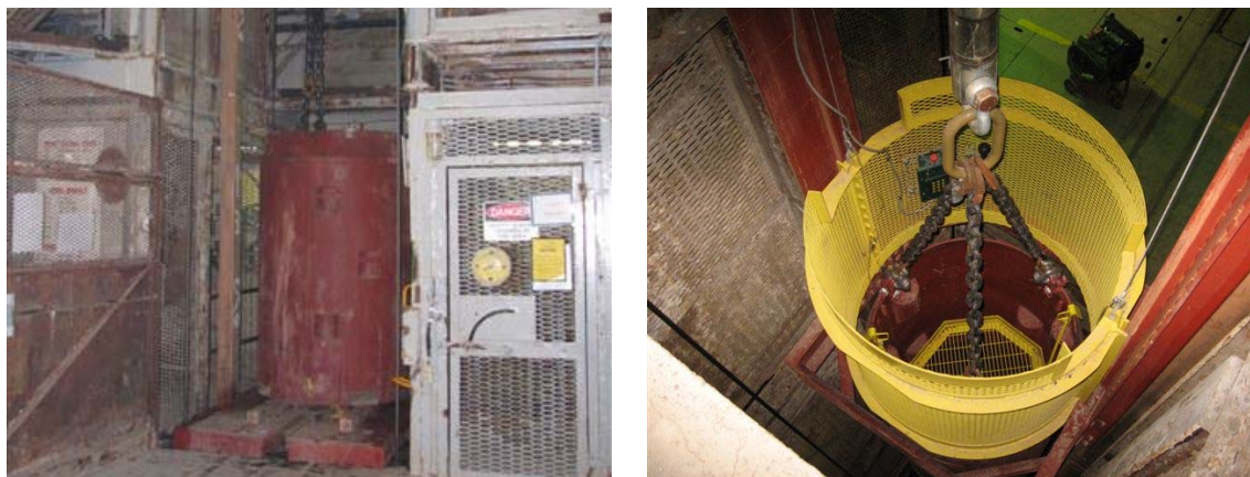
Figure 5. Sinking bucket and bird cage.
