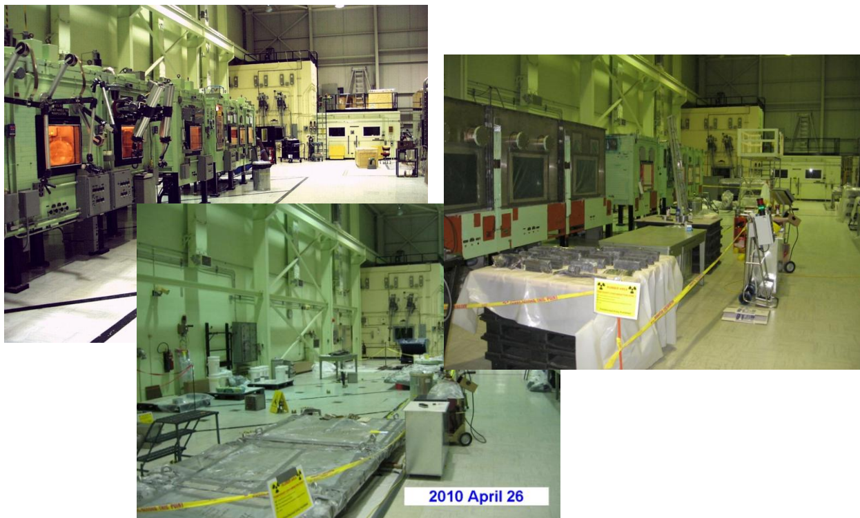
Figure 5. Decommissioning of Warm Cells 14-18 in the WL Shielded Facilities (before, during and after).
