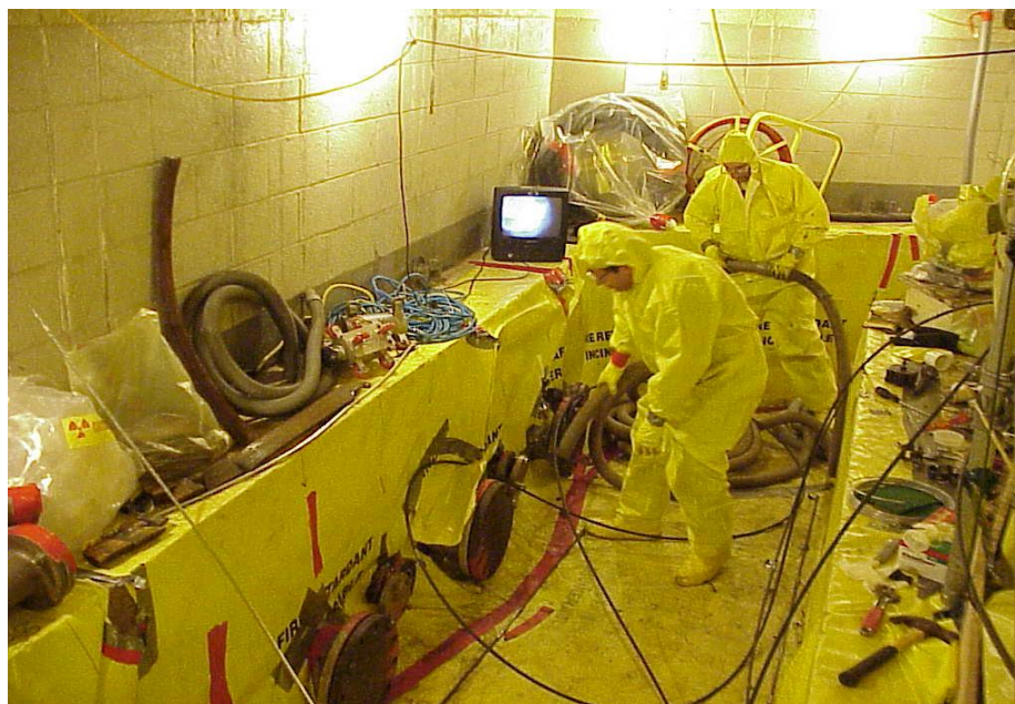
Figure 2. Workers Cleaning Embedded Piping
