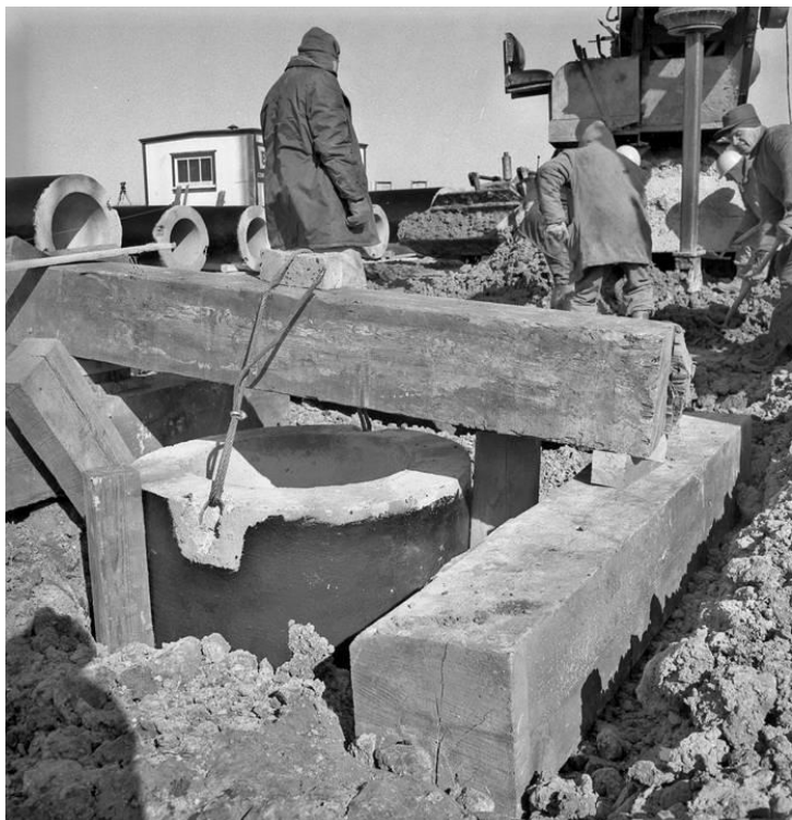
Figure 2. Installation of an early standpipe (circa 1966). Note work in the background on augering another standpipe hole.
