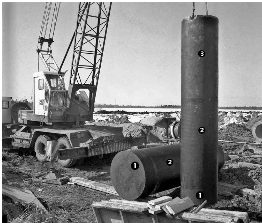
Figure 1. Standpipe sections 1: base; 2 and 3: unlined pipe (circa 1966).
