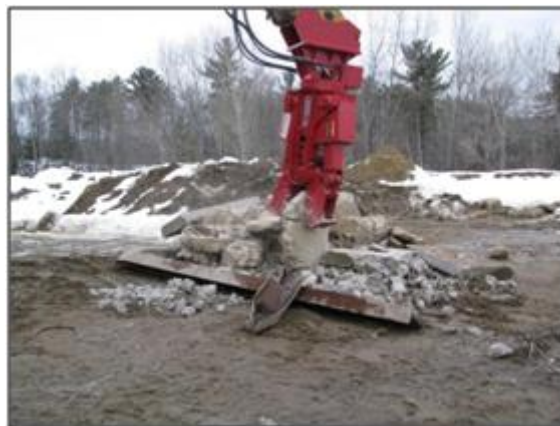
Figure 1. Multi-Processor with Pulverizer attached to CRL excavator
