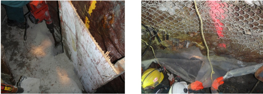
Figure 7. Seepage control measures, cribbing (left) and water collection (right).
