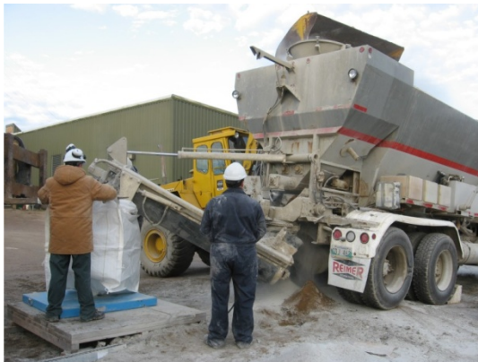
Figure 6. Clay mixing and compaction.
