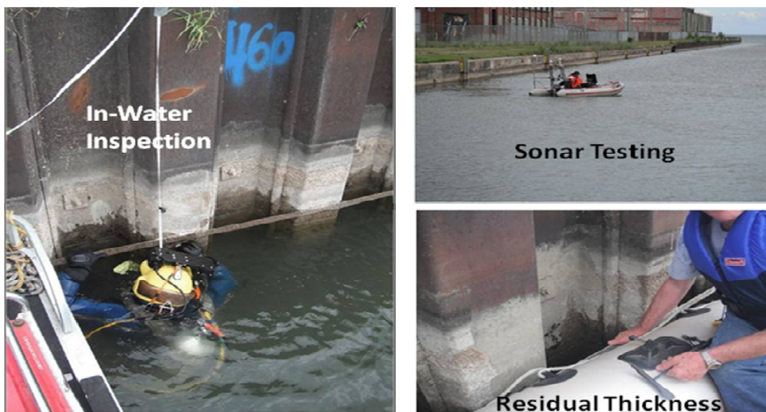
Figure 9: Harbour Wall Condition Assessment Activities
