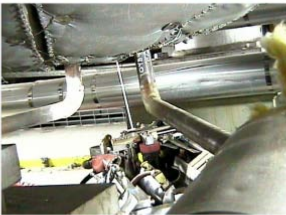
Fig. 13. Pipe Removal (Freeze and Cut) Robot in position.
