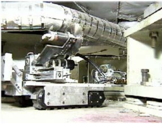
Fig. 11. Insulation Removal Robot making circumferential cut.
