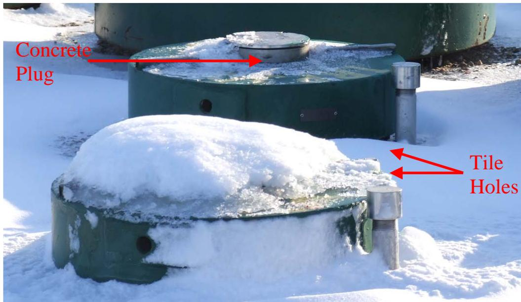
Figure 1 Tile holes in Waste Management Area (WMA)
