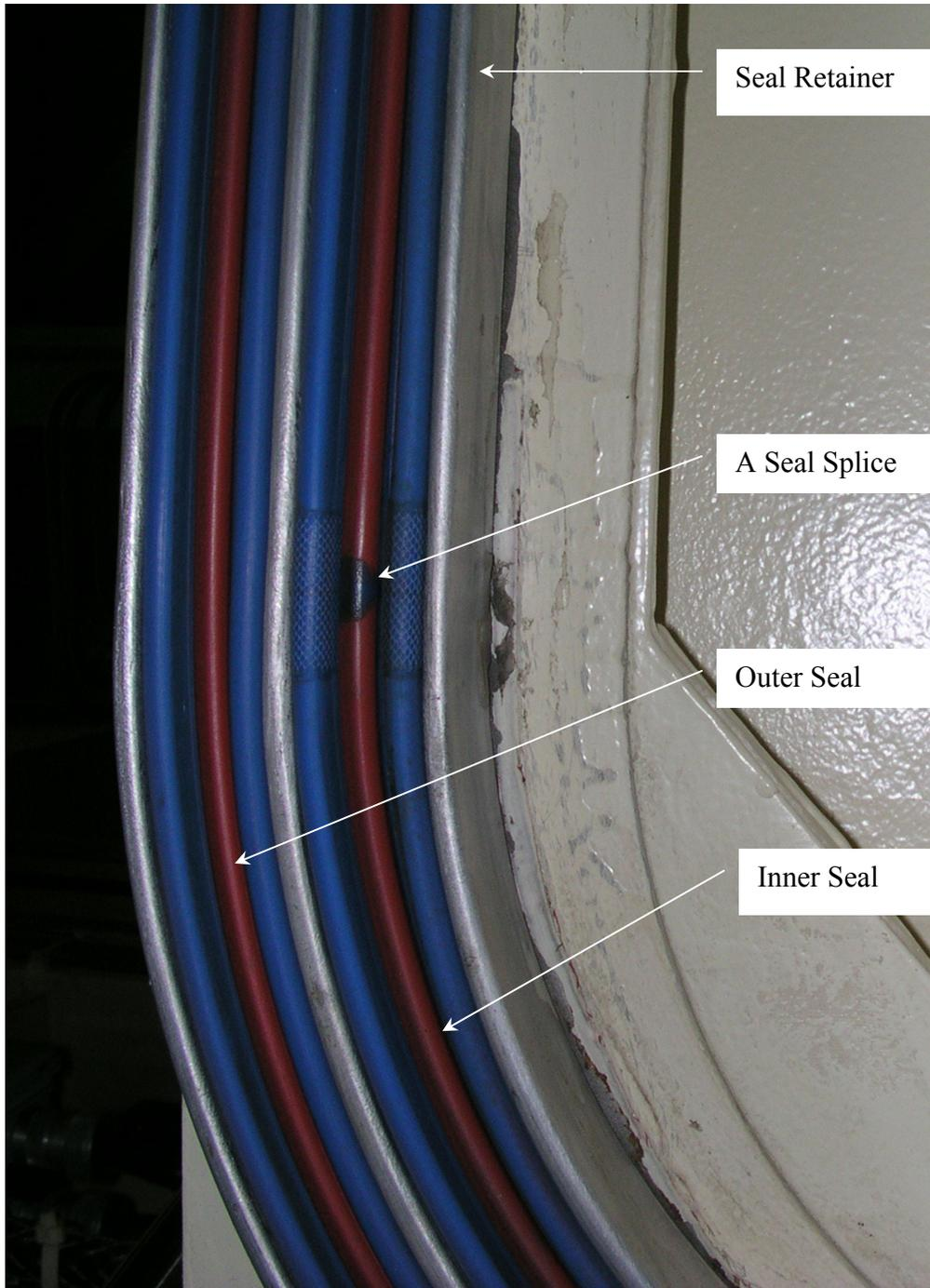
Figure 4: One Corner of a Personnel Door Showing DSA1 Seals
