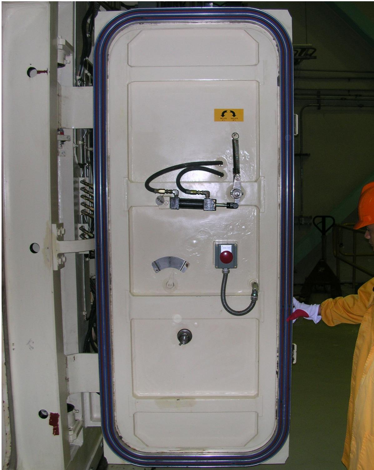
Figure 3: DSA1 Seals Installed in a Personnel Door of the Qinshan Equipment Airlock
