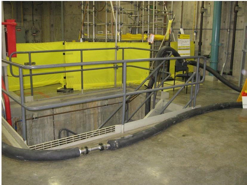
**Figure 6: Hoses Run Up the Railing and Down the Stairs to Simulate the Vent Riser**
