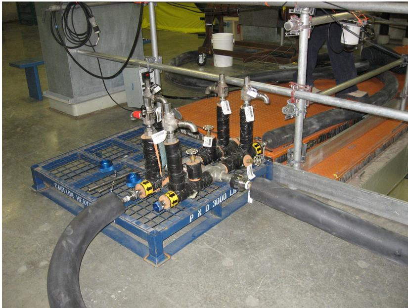
**Figure 7: Header at 92.5 m Elevation, Supplying Single Hoses to both Freeze Jackets**
