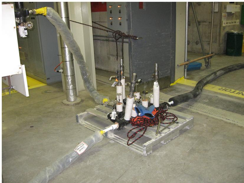
**Figure 4: Tanker and TK1 Connected to a Single Header in the Simplified Arrangement**
