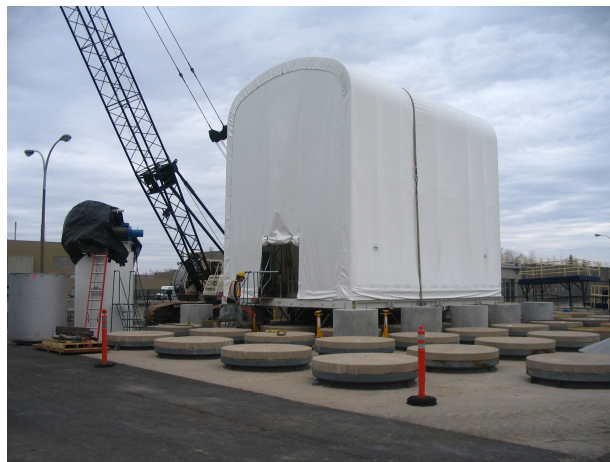
Figure 2: Construction Island Showing the Enclosed Work Platform, Crawler Type Crane, Over-Pack and IC-18s
