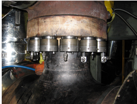
Figure 2: Hand tighten onto stud
