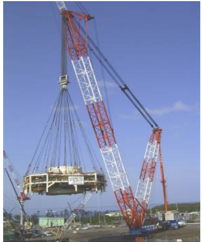
Figure 1 RCCV Upper Drywell Module
