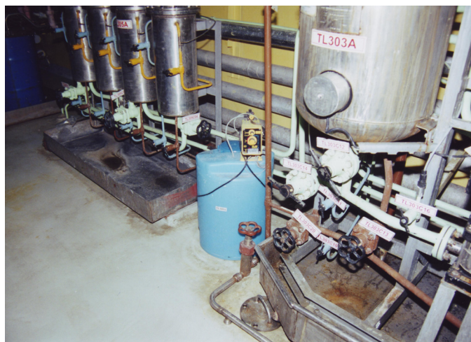
Figure 5: Liquid Radioactive Waste Management (Reverse Osmosis Equipment)
