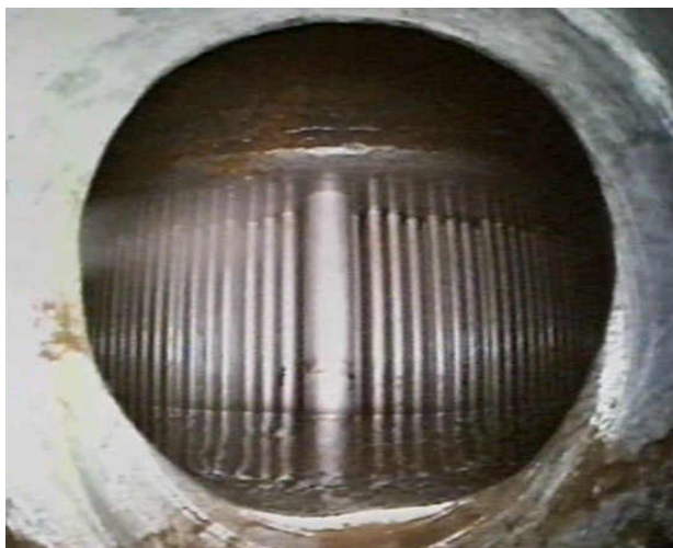
Figure 2: Cleanliness of Secondary Side Internals
