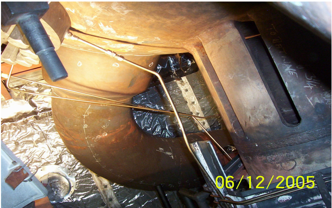
Figure 4 – Piping walkdown (inspection sites are marked on the piping)
