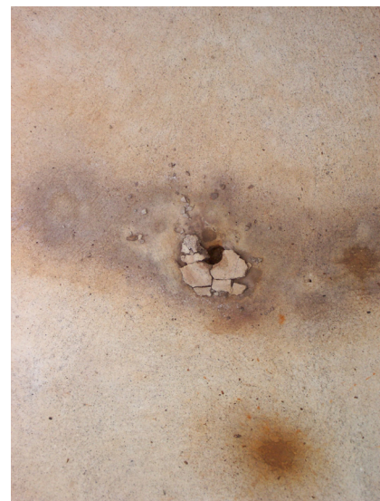
Figure 2 Example of shield-plug lifting insert deterioration
