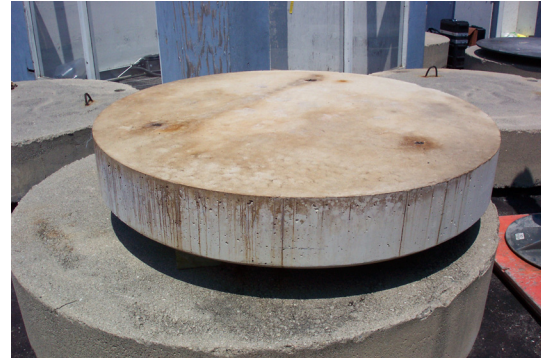
Figure 3 Another example of shield-plug lifting insert deterioration
