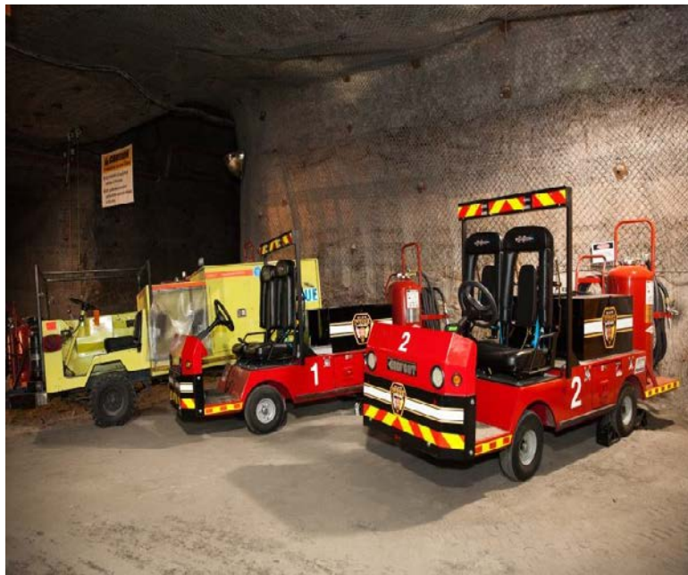
Figure 3. New fire suppression and emergency response equipment in the underground
