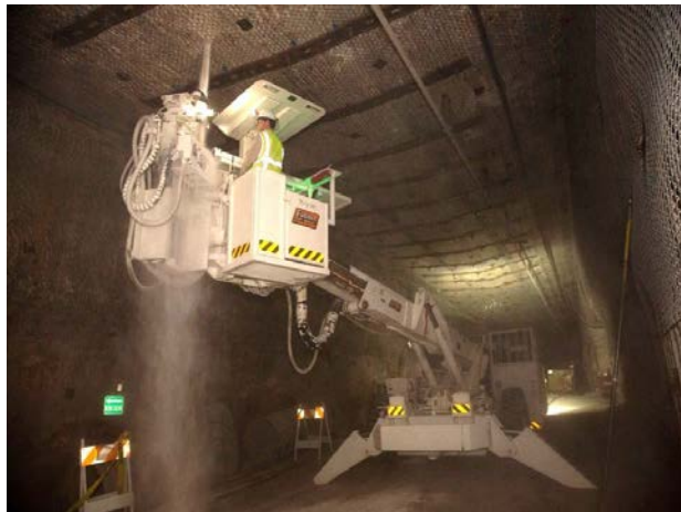
Figure 4. A hybrid (diesel and electric) bolting machine conserves breathable air while bolting, allowing more simultaneous underground recovery activity
