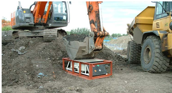
Figure 6 The Gamma Excavation Monitor System
