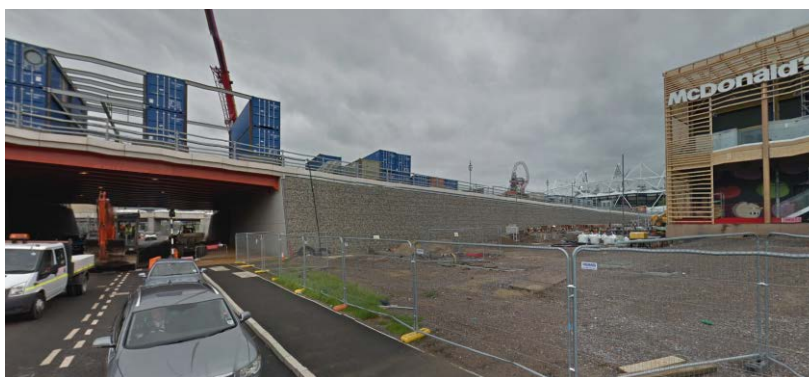
Figure 9 The completed Bridge Abutment with Disposal Cell
