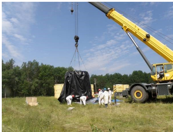
Figure 6 Preparations: spreading of suspect soil (left), relocation of NRX stack pieces (right)
