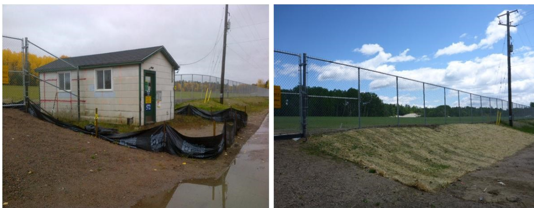
Figure 13 Gate house before and after removal
