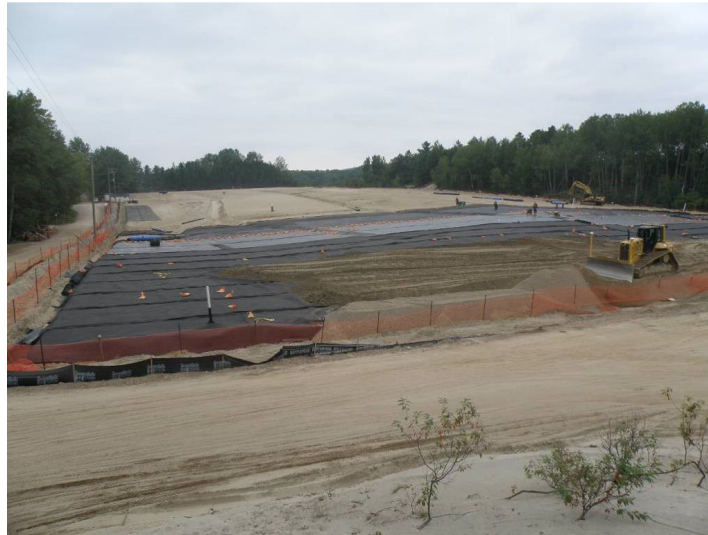
Figure 10 WMA C during cover installation (2013 August)
