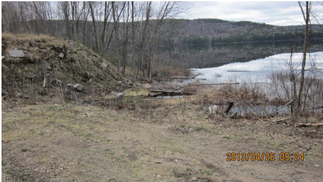
Figure 5: South side of Dump #2 as it appeared in 2013 April
