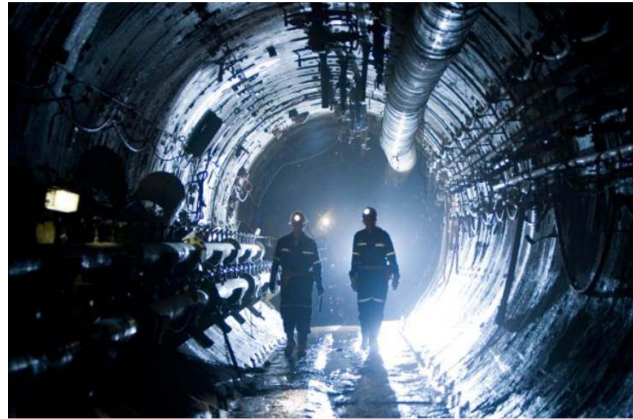
Figure 8. Concrete segment lined tunnel with freeze piping
