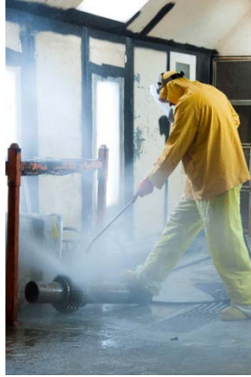
Figure 10 High Pressure water/Low pressure steam with chemistry, a basic decontamination process.
