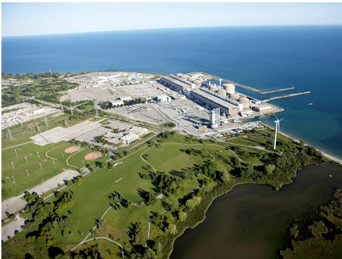
Figure 1 Aerial view of the Pickering Nuclear site.
