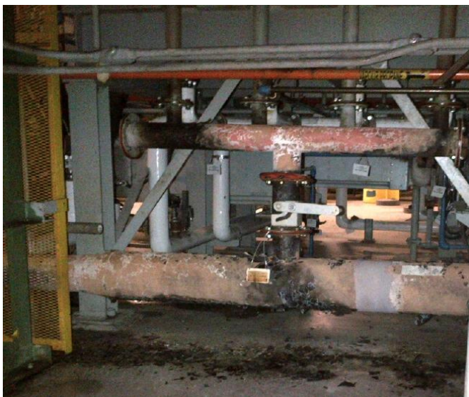
Figure 6: Damage to underfire air duct
