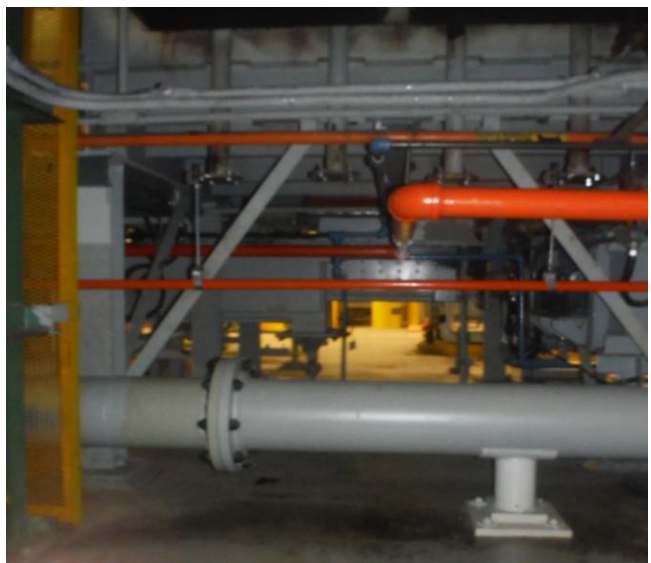
Figure 7 post-mod: underfire air tubes capped
