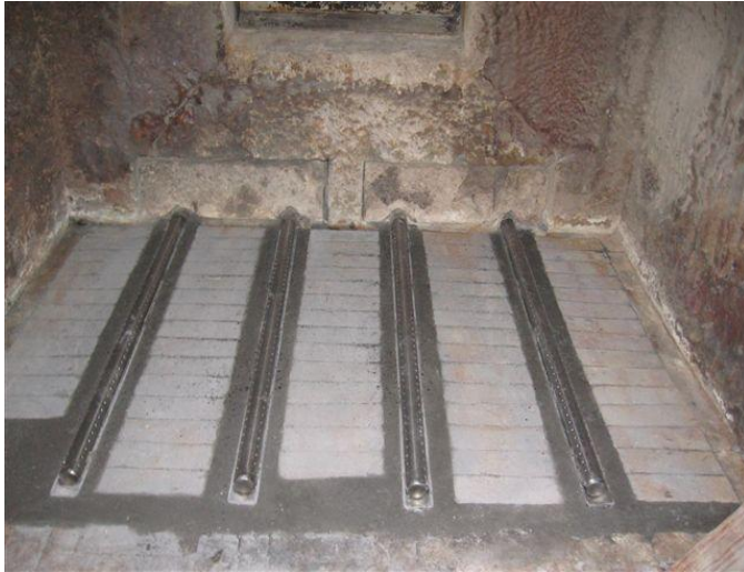
Figure 4: pre-modification: underfire air tubes Figure 5: post-modification: solid hearth
