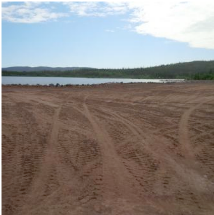
Photo 2: Cover on mine tailings at Lorado before final grading and seeding in 2015
