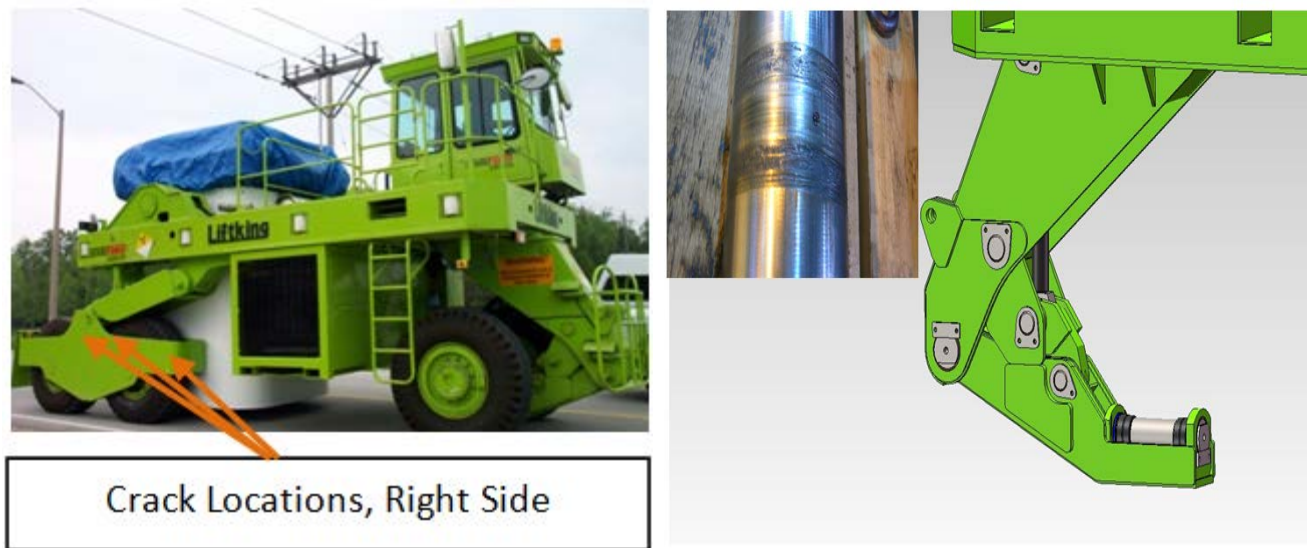
Figure 5 (a) walking beam cracked welds in cross members (b) damaged lift joint pin
