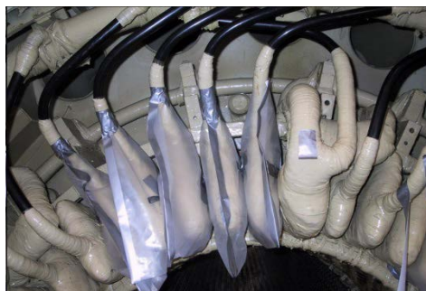
Figure 4: Stator Winding Leak Test Using Event Bagging (Bags shown on left hand side)
