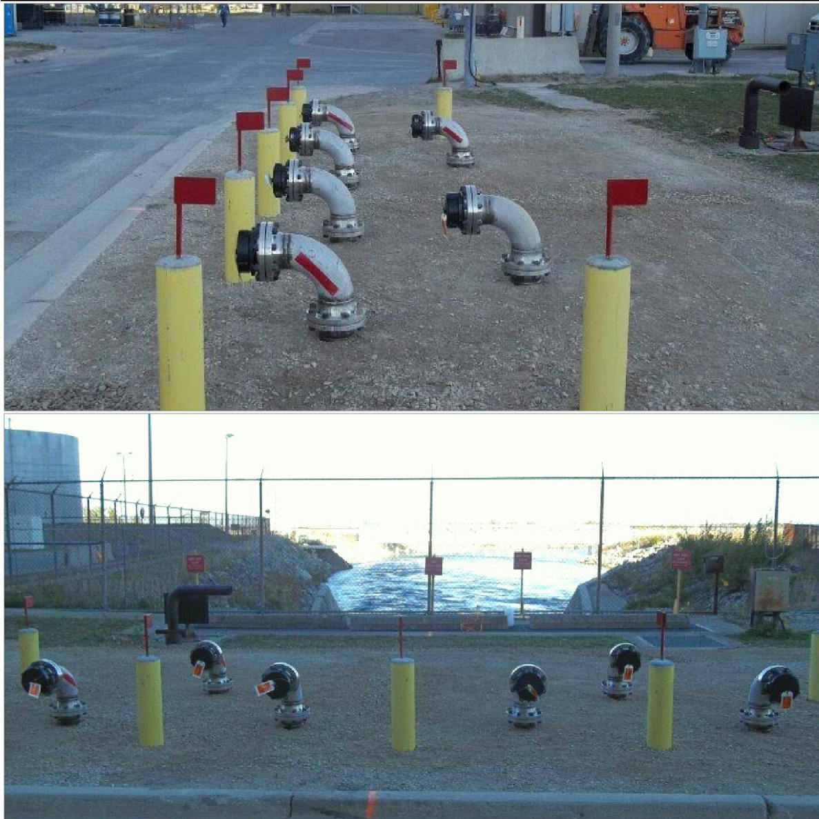
Figure 3 Installed Emergency Water Dry Hydrants
