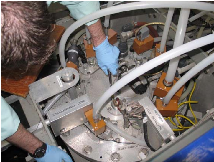
Figure 7 Commissioning of the Replacement Cd-Emitter SPD
