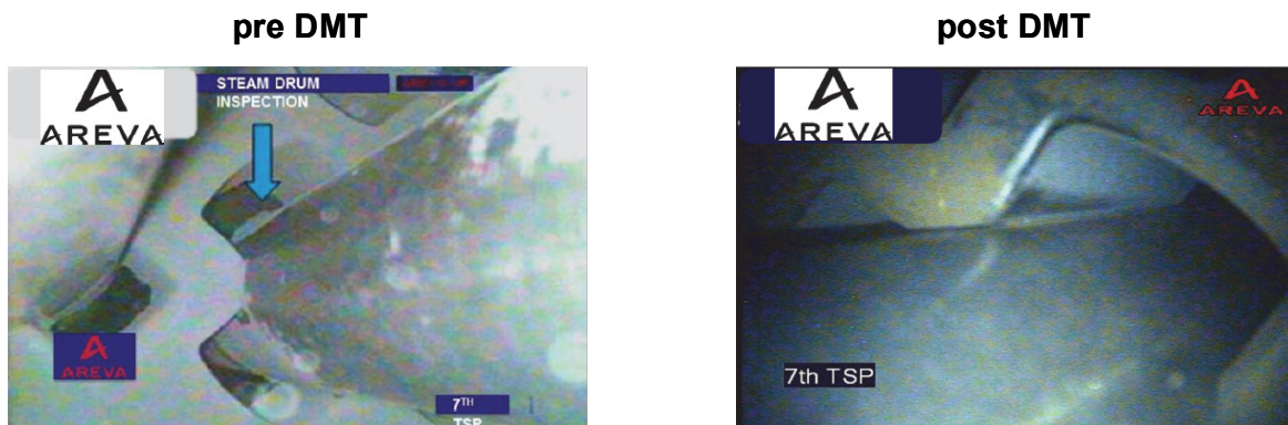
Figure 10. Visual inspection results prior and after application of AREVA's DMT process
