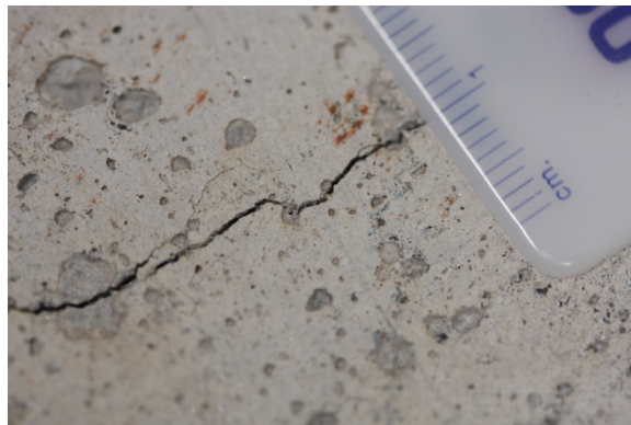
Figure 8: Image of the crack that occurred during the 820 °C curing process of the ceramic.
