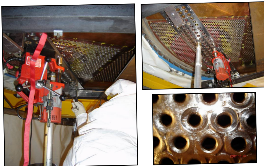
Figure 11 : Semi-Auto End Facing Tool and example of repaired tube ends before final boring
