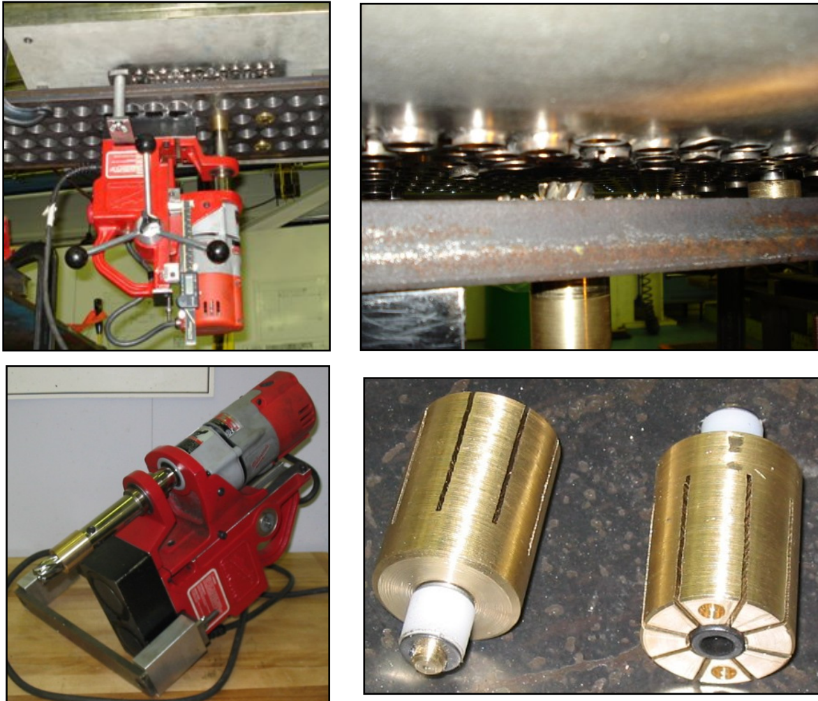
Figure 9 : Magnetic based drill on the mock-up in the shop and the brass bushings used for the alignment of the plate
