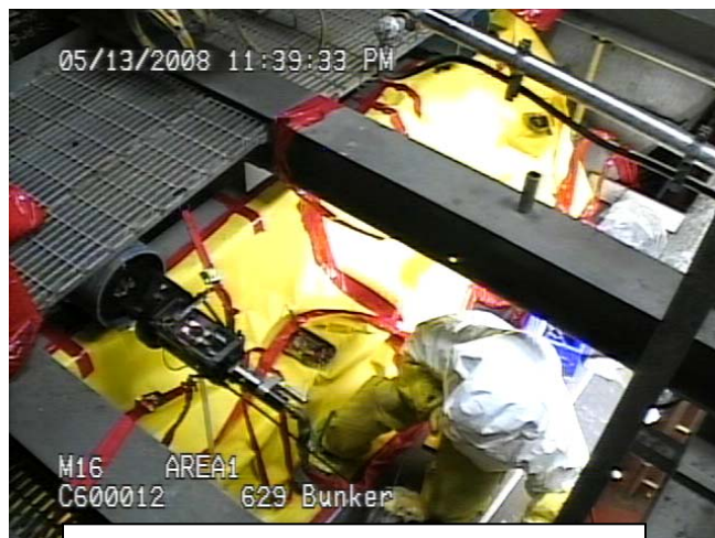
Tool installation at Bruce Power unit 5
