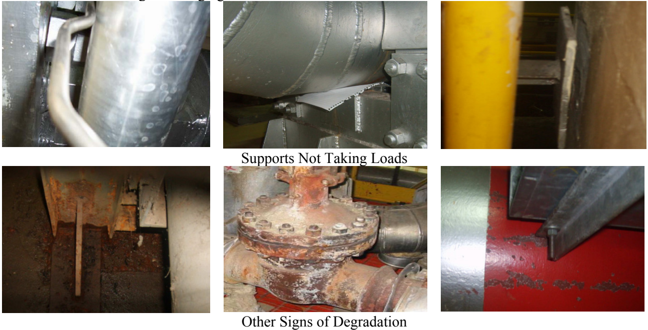
Figure 3 Pictures Showing Condition of Select Nuclear Pipelines
