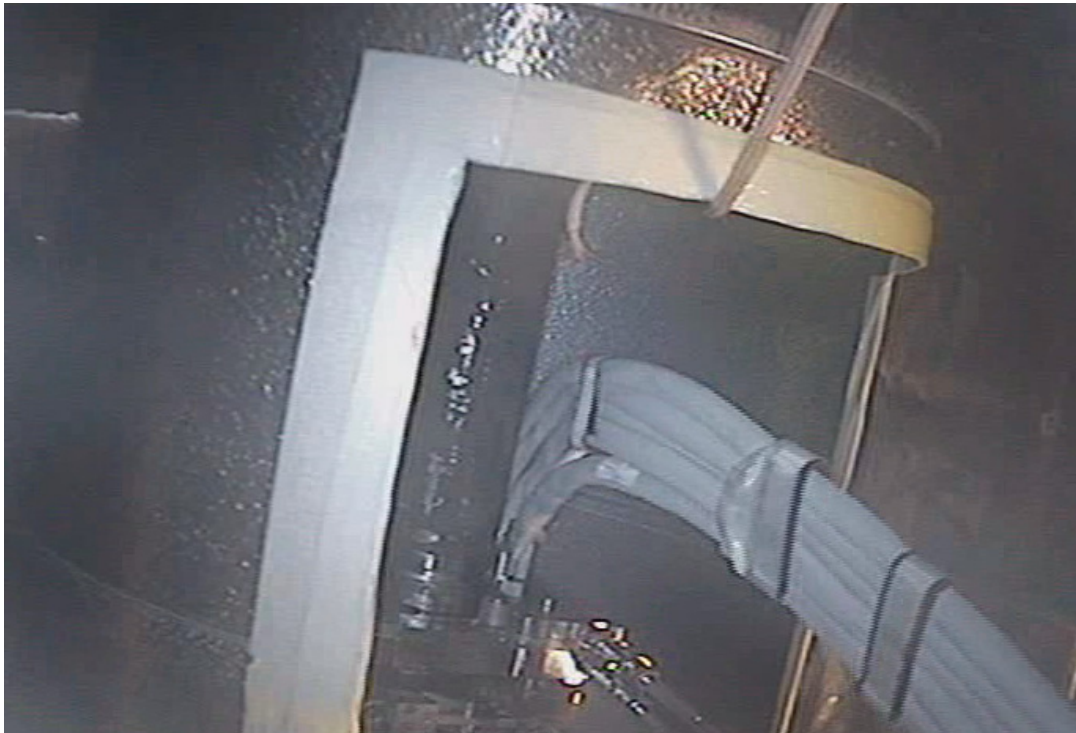
Figure 7 - Draft Reduction System, initial installation.
