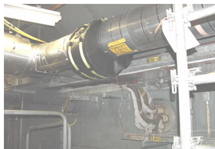
Figure 8. ECI Hot Spot Water Bag Shielding
