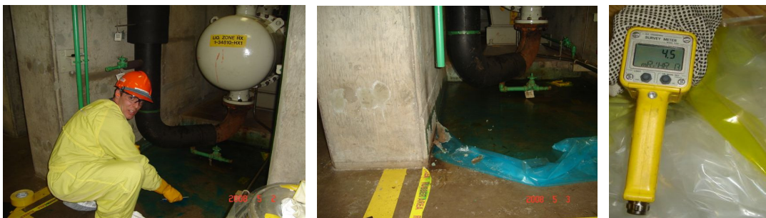
Figure 10. Decontamination Using Strippable Paint
