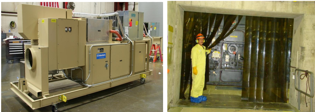
Figure 14. Use of Munter Dryer and Plastic Curtain to Reduce and Contain Tritium
