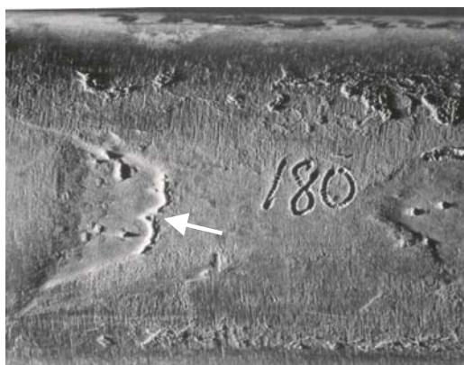
Cleaned surface at the affected region
