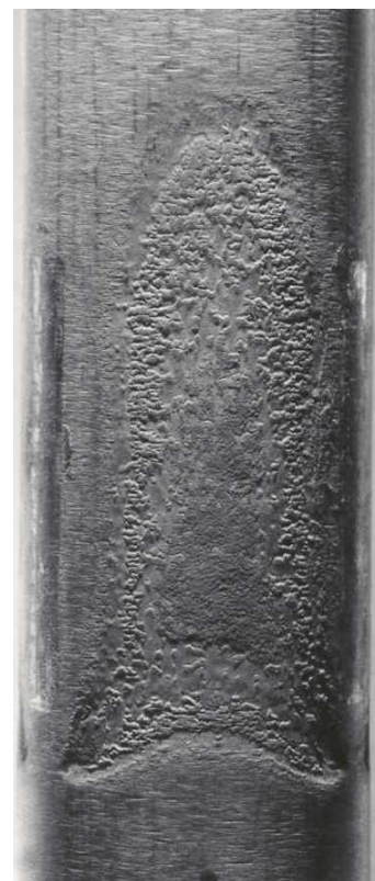
Fully developed erosion corrosion feature at 8 th Support
