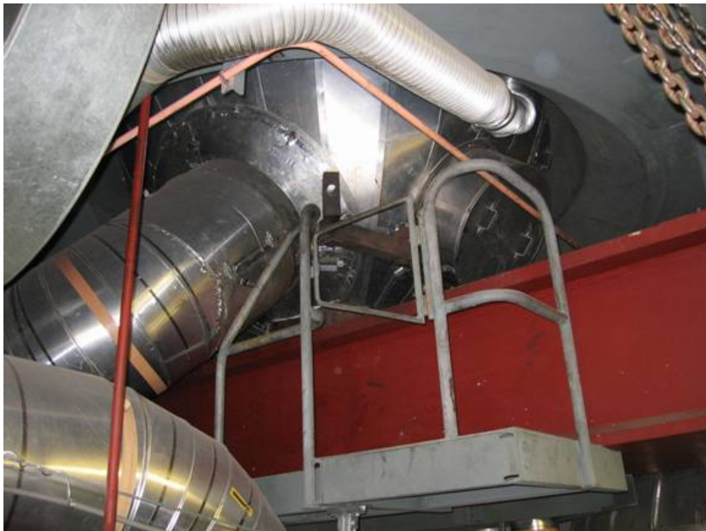
Figure 5-13: Vault PHT Piping & Support Arrangement
