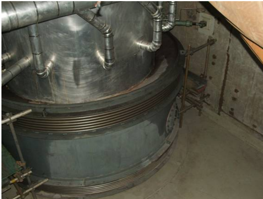
Figure 5-4: View Inside Boiler Room Above Vault Showing Containment Expansion Joint & Blow Down Lines
