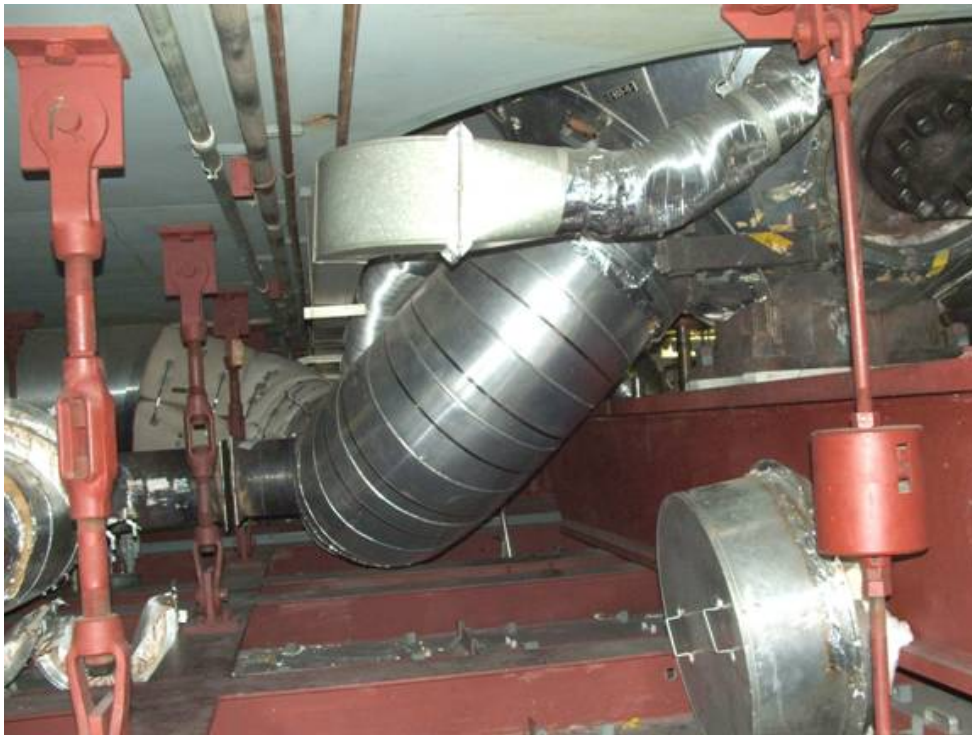
Figure 5-11: Vault Showing Trapeze Support, PHT Outlet Piping & Part of Balance Line
