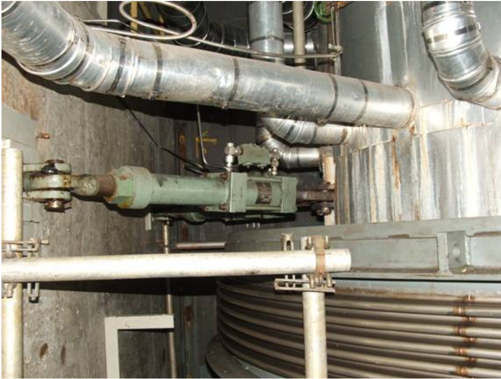
Figure 5-2: Boiler Room, top of the Containments Seal Assembly & Seismic Restraint
