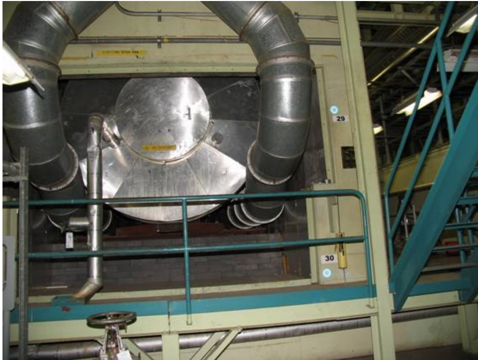
Figure 5-10: Steam Drum Face Showing Cooling Ducts
