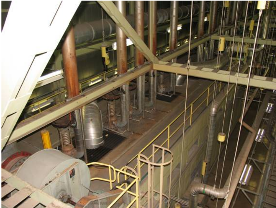
Figure 5-8: View of Top of Steam Drum Enclosure Showing MSSVs & Cooling Fan
