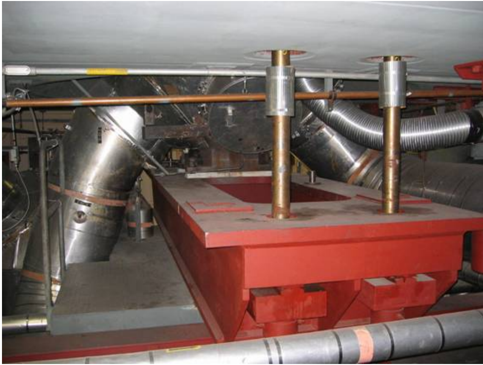
Figure 5-14: Vault PHT Inlet & Supporting (Trapeze) Arrangement
